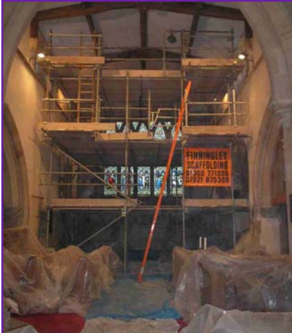
Scaffolding in the church ready for work to start
